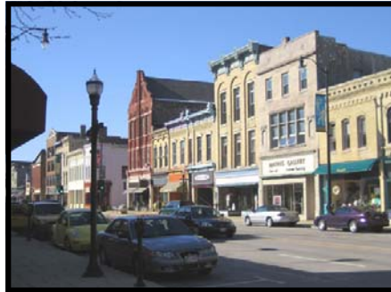
Appropriate. Special features enhance the pedestrian experience and a scale that fits the historic structure of downtown.
